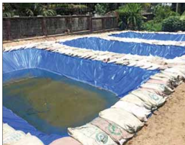
Fig. 57b Nursery pond with lining (8 x 4m)
